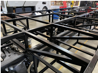
More Steel in the Sub-Floor forming a Strong Foundation.
