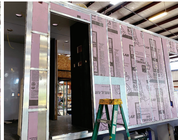
3" Headers & Slide Openings Wall Studs 16" On Center.
