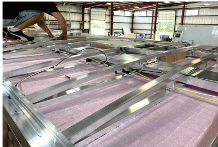
Strong Aluminum Roof Trusses Every 16" On Center.
